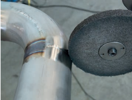
Removing welding discoloration.
